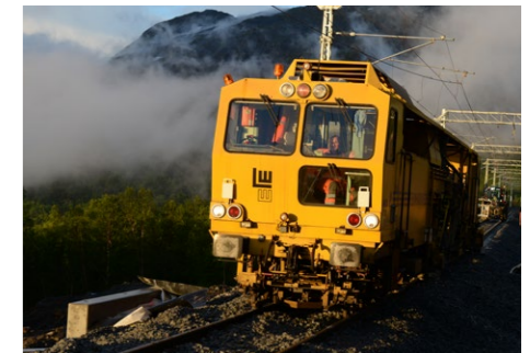
Track construction in Norway
