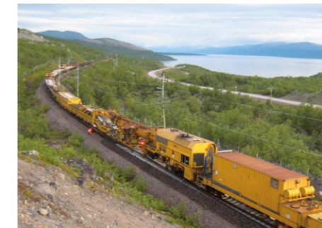
Track construction in Sweden
