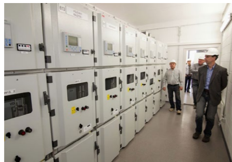
Power supply / network construction in Estonia
